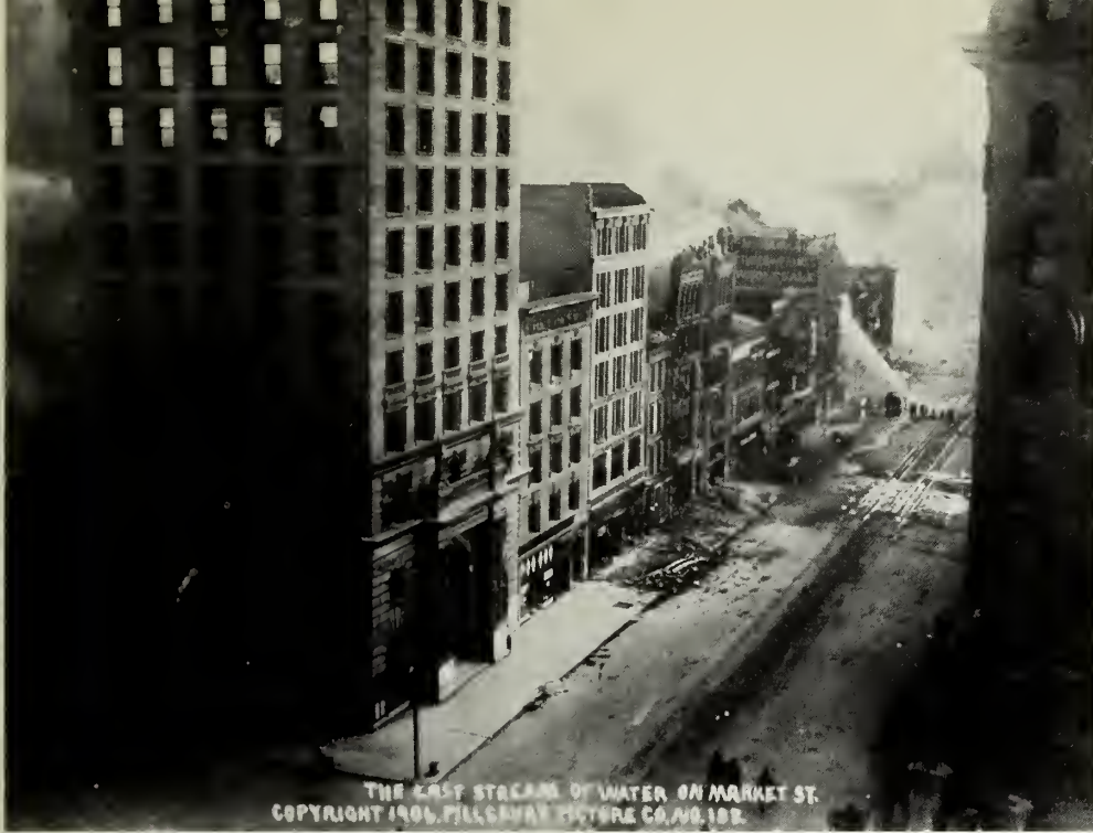
Plate 51: Running Out of Water . . . Cisterns allowed firemen to put up a fight along the Market frontage of Central Block 1—but there was too much fire and not enough water. (Society of Calif. Pioneers)
